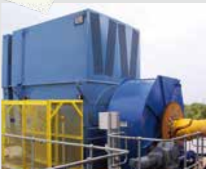
4,476 kW, 11,000 V, 12P, frame 1000 (MGF) HITCHIN – LYNX - England
