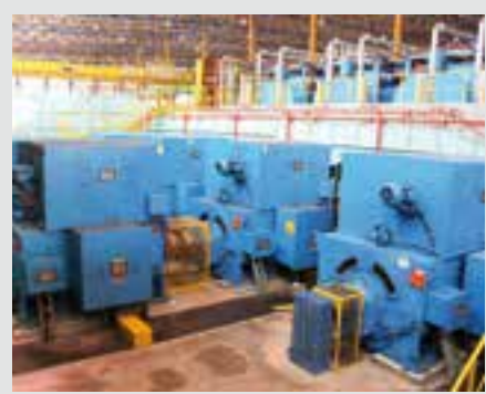
7XSDL800, 3,000 kW, 6P, B3R Laminator Motors, VEGA DO SUL (Arcelor Group) - Brazil
